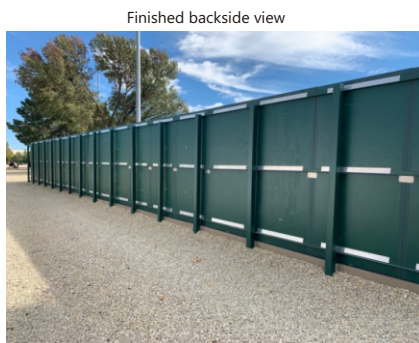
Finished backside view
